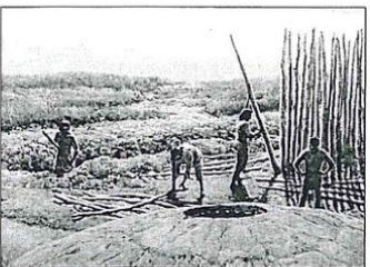
Ten people building a palisade (wooden fence) and digging a ditch
